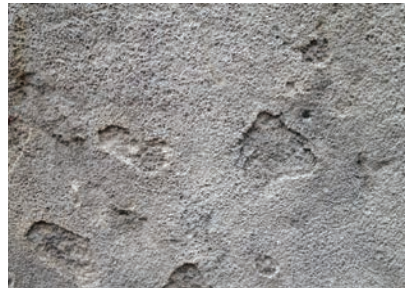
Freeze-thaw spalling
